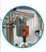
The vacuum protection valve safely prevents sap overflow in your moisture trap or your vacuum pump without shutting vacuum down.
