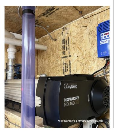
Being a sugarmaker on top of having a full-time job is tough. I needed equipment that was dependable. My biggest concern was getting a vacuum pump that would be reliable, capable of high vacuum, and be cost effective to run. I did not want to deal with oil cooled pumps because of high maintenance and moisture contaminating the oil.
